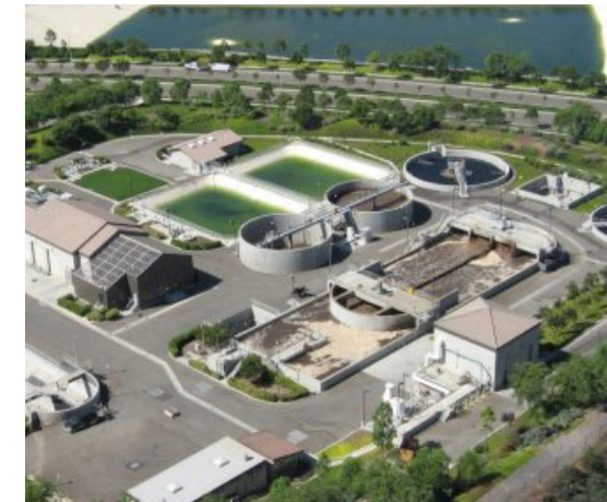
4S Ranch Water Reclamation Facility
